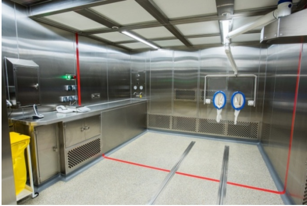
Rigid Barrier Screen within Facility
